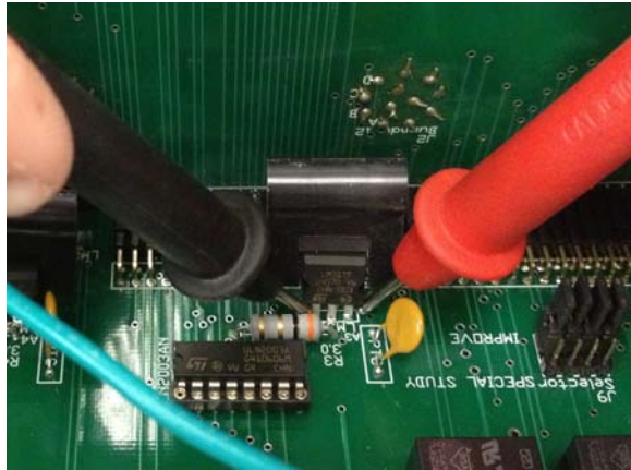
Figure 4. Checking Voltage Regulator
