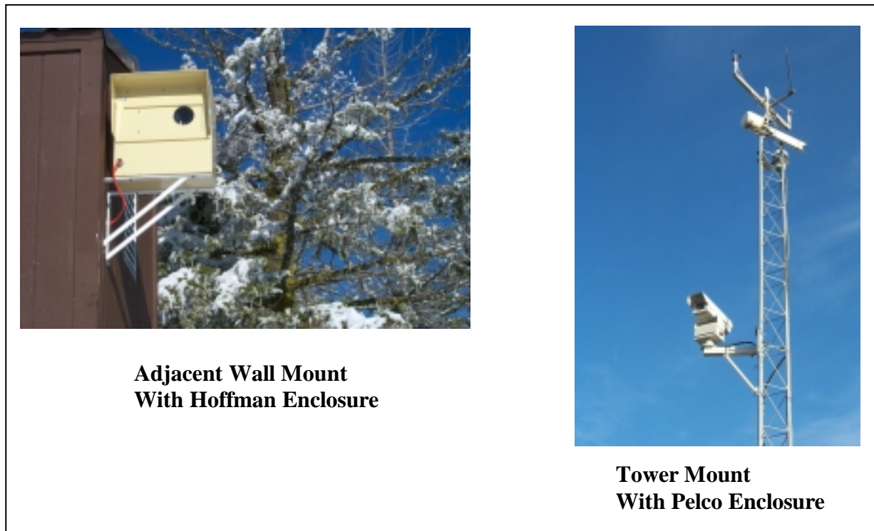
Figure 4-5. Example Camera Enclosure Mounting Types Using Mounting Brackets.
